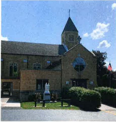
Oakfield Site 56 Maple Ave., Oakfield
